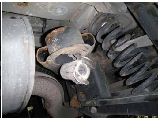
Same salt corrosion failure, different view.
